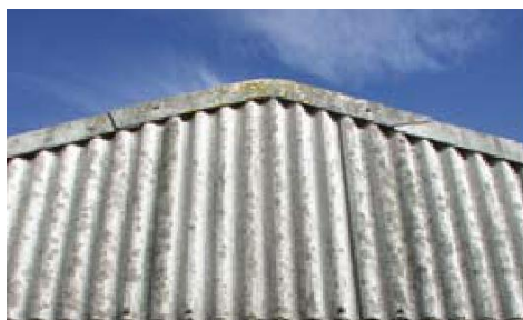
Asbestos cement wall cladding
